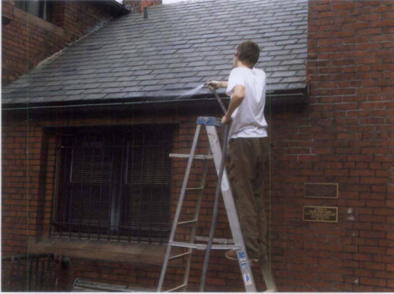
Figure 3. Keeping gutters clean of debris can be one of the most important cyclical maintenance activities. On this small one-story addition, a garden hose is being used to flush out the trough to ensure that the gutter and downspouts are unobstructed. Gutters on most small and medium size buildings can be reached with an extension ladder and a garden hose. Photo: Bryan Blundell.
