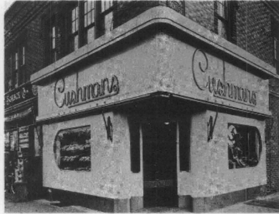
Figure 4. This storefront in New York City designed by Raymond Loewy typifies the streamlined look of the 1930's. Added to an earlier building, the front utilizes glass, stainless steel and neon to make a modern statement. This is a good example of a later storefront which has acquired significance and should be retained in any rehabilitation.
