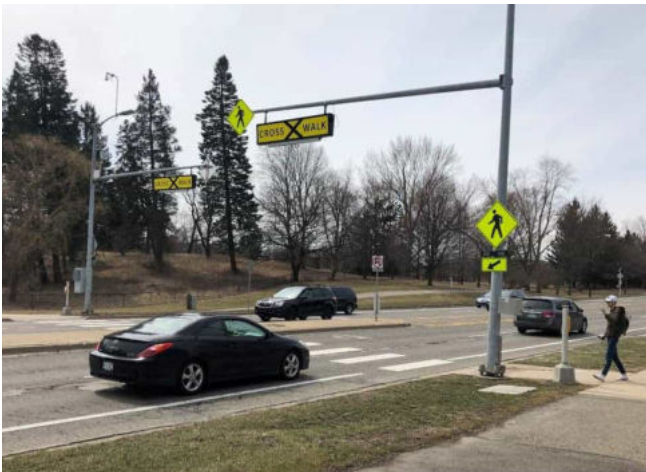
Rectangular Rapid Flashing Beacons (RRFBs) can be utilized at midblock crossings to improve safety for pedestrian crossings.
