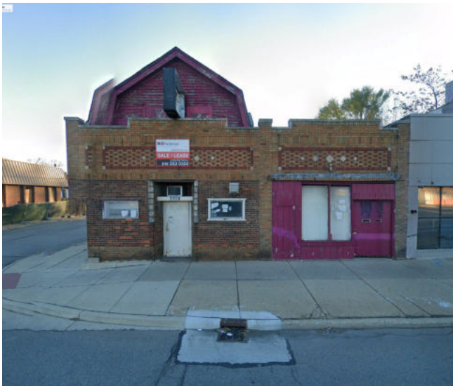
Existing vacant building along the corridor
