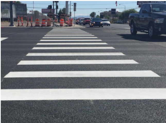
'Piano bar' crosswalk striping enhances visibility of pedestrian crossings.
