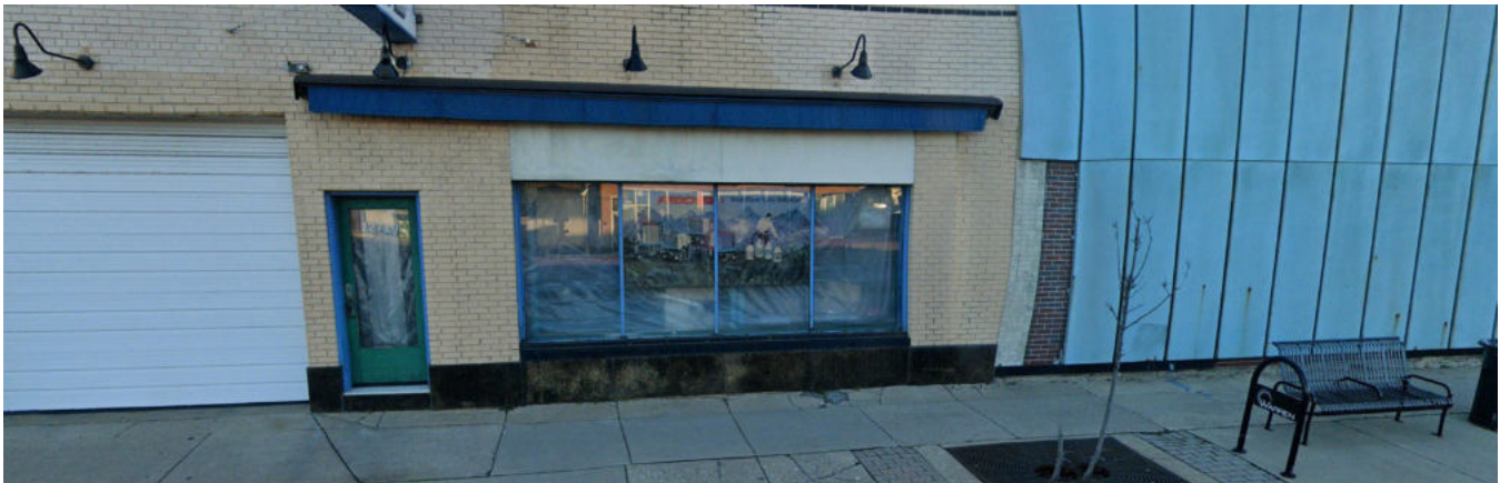
A vacant commercial property along Van Dyke Avenue.
