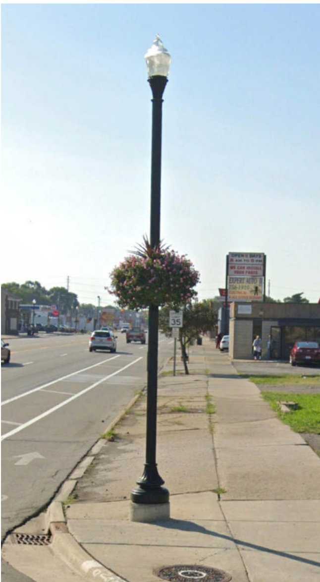
Existing post-top lighting along the corridor is recommended to be expanded or installed at shorter intervals to improve pedestrian-scale lighting along Van Dyke Avenue.
