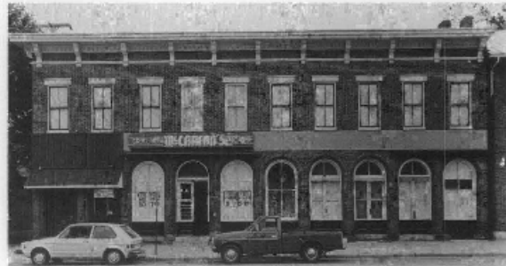
Figure 5. In some cases, as in the storefront on the extreme left, it is a simple matter to determine original appearance by looking at neighboring storefronts. Removal of the board and batten fasciaboard, pent roof, and "colonial" style door, all of which could be undertaken at minimal cost, would restore the original proportions and lines of the building. Photo: Day Johnston
