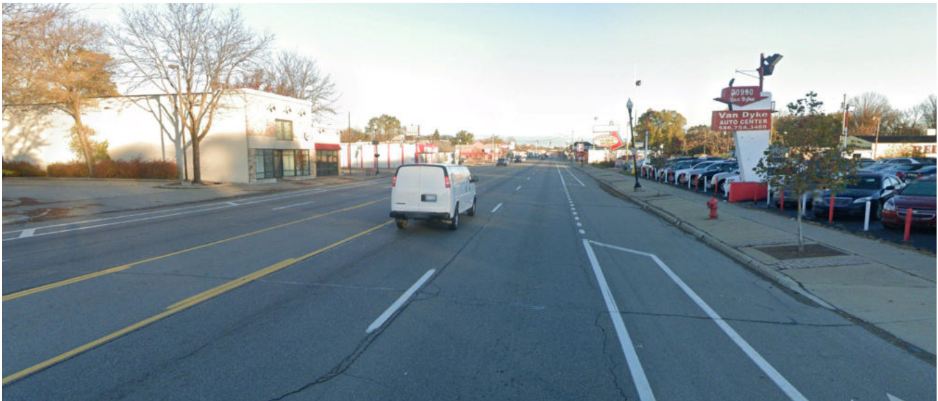
Van Dyke Avenue at Fisher Avenue northbound shows the current character of the corridor as vehicular-centric.
