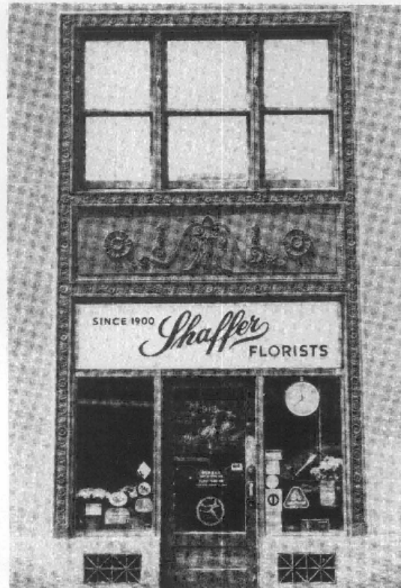
Figure 7. Part of a large office building constructed in Washington, D.C. in 1928, this finely detailed bronze storefront is typical of many constructed during this period. It should be noted that the original grilles, spandrel panel and window above are all intact. Photo: David W. Look, AIA
