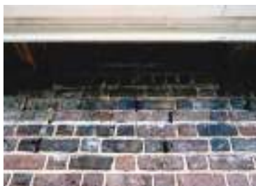
Careful examination of the masonry reveals different periods of construction and repair through the composition and detailing of bricks and mortar. Depending on location, the vertical open joints may indicate the location of nailing blocks for decorative trim or weeps for drainage. Photo: Travis C. McDonald, Jr.
