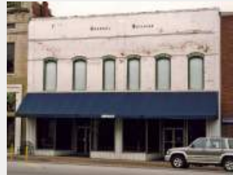
The photograph above shows the building described in the sample application prior to the rehabilitation work. Below left, the building is shown after its successful rehabilitation.
