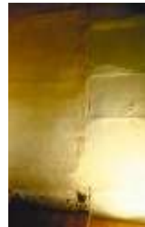
Raking light is used to show irregularities on flat surfaces. Patches, repairs, and alterations can then be mapped by the shadows or ghosts they cast. Photo: Travis C. McDonald, Jr.
