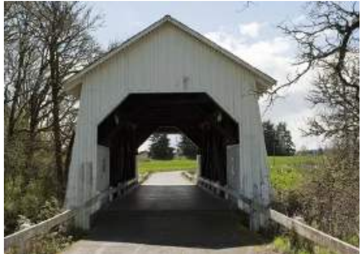
Irish Bend Covered Bridge No. 14169, Covallis, Oregon
