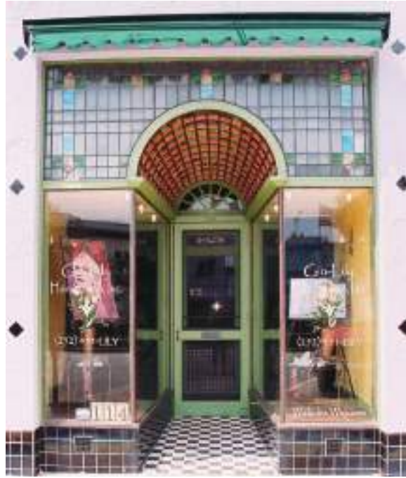
114 NW Main Street, Rocky Mount, North Carolina (1928). Photograph: William Ferguson.
