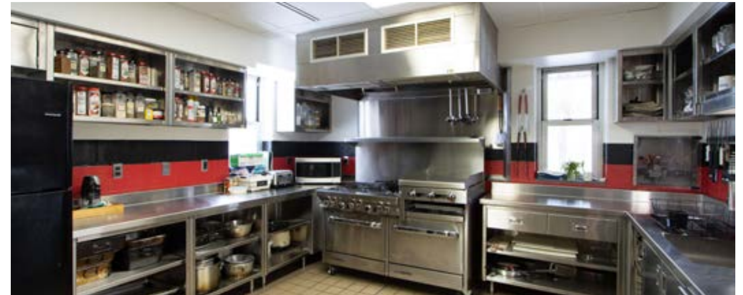
(Above: Newly renovated kitchen at Warren Fire Station 2 on Schoenherr between Stephens and 9 Mile)
