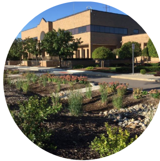
Bioswale installation at Clinton Township Civic Center
